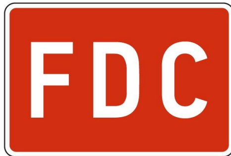
Photo 5 – Fire Department Connection Sign
